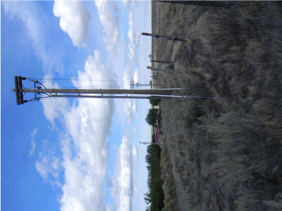
View of pole with residence in background
